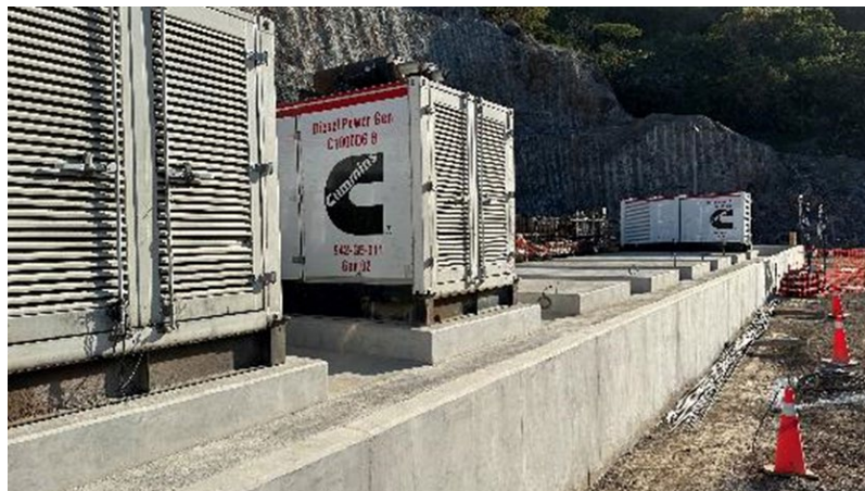
Back-up generator farm outside South Portal Upper
