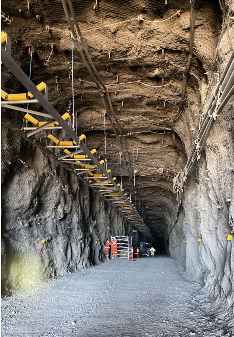
Conveyor table installation
