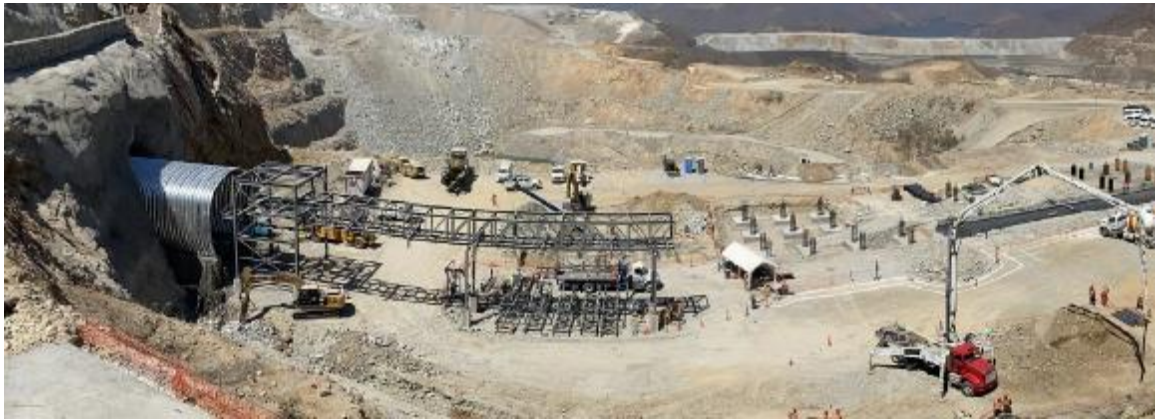
Steel infrastructure for monorail load-out
