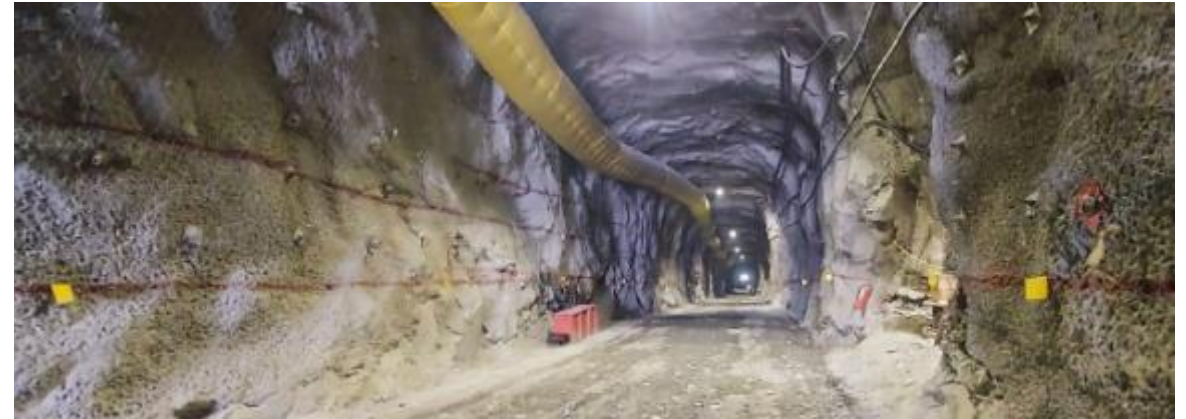
Guajes tunnel advanced ~300 metres
