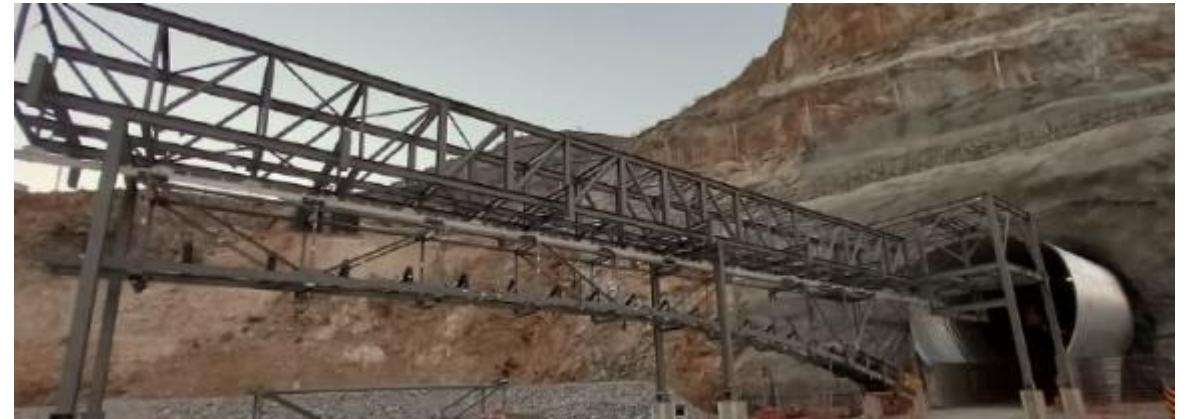
Installation of bridge conveyor
