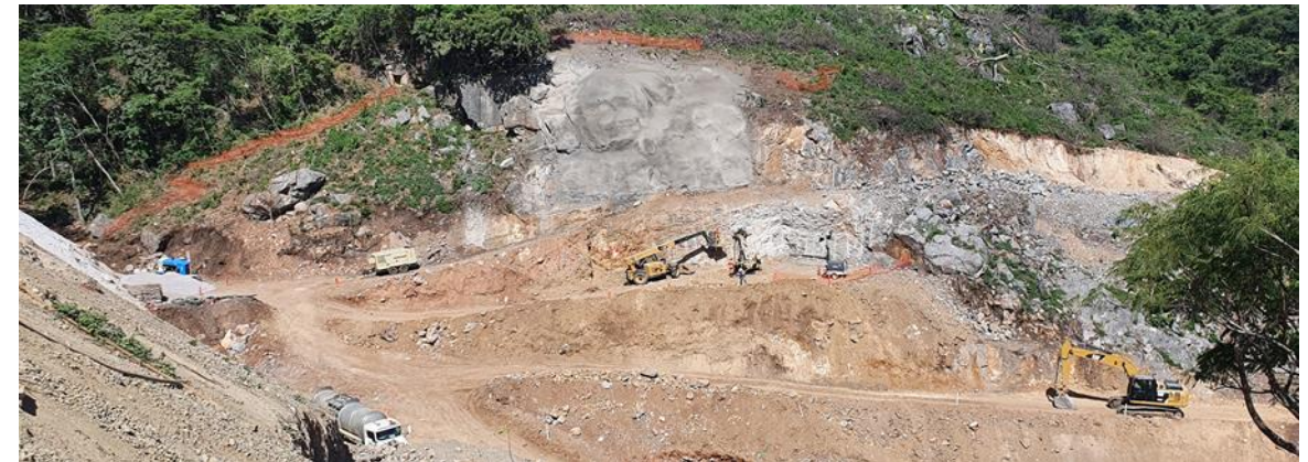
Prep of South Portal Upper well underway
