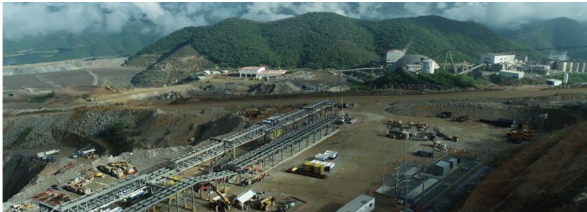
Overhead shot of loadout facility and plant
