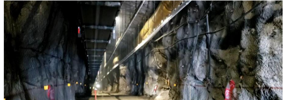
Total Guajes tunnel development of 450 m
