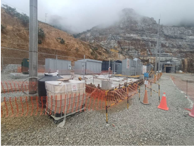
Preparation of pad for paste plant
