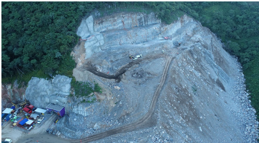
Preparation of pad for paste plant
