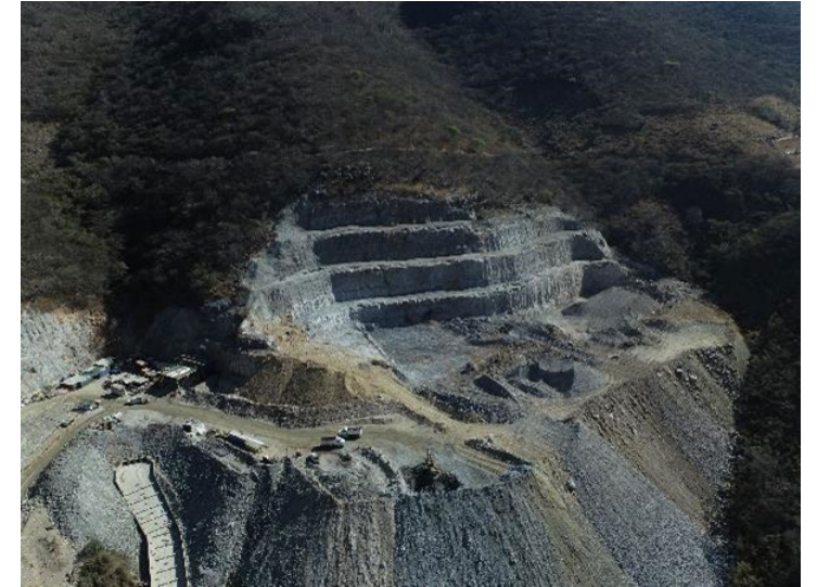
Paste plant pad preparation
