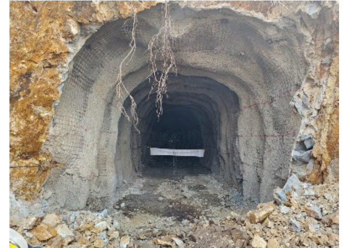
West Adit Vent tunnel breakthrough
