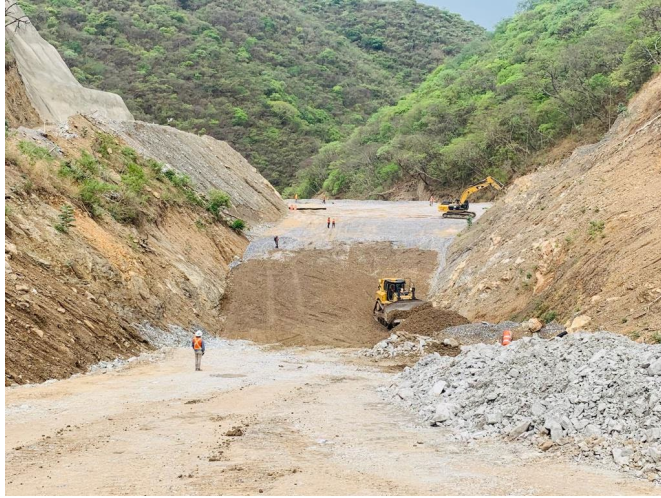
Work continuing for sedimentation pond
