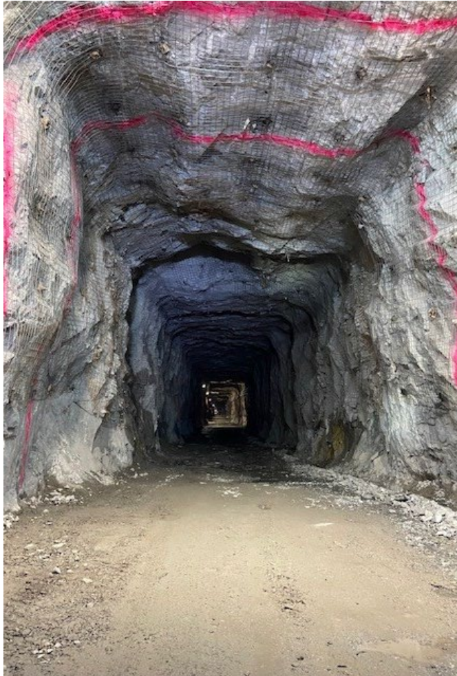
Guajes Tunnel breakthrough
