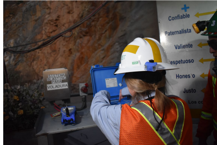
CEO Jody Kuzenko initiating final blast for Tunnel breakthrough
