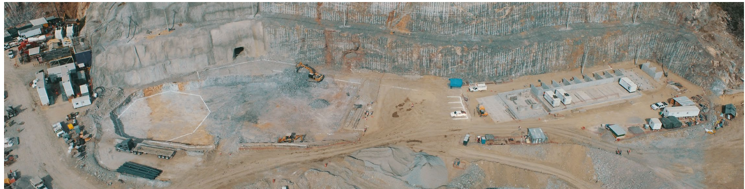
Foundations for paste plant outside of South Portal Upper
