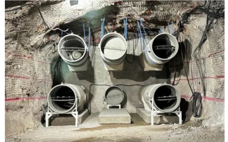
West adit fan installation for underground ventilation
