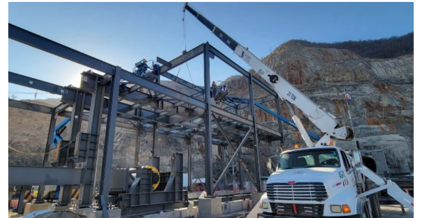
Steel erection for Guajes conveyor head
