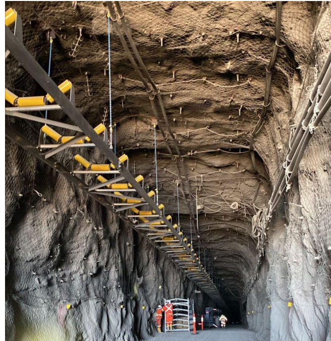
Conveyor table installation
