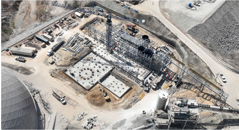
Surface construction at flotation circuit
