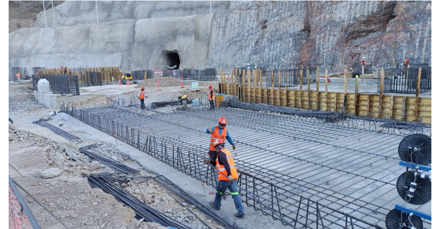
Concrete work for paste plant
