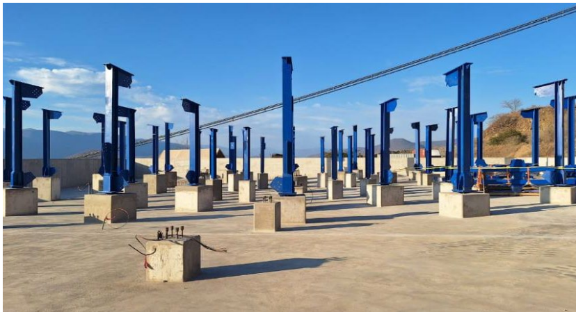
Steel erection at Guajes thickener
