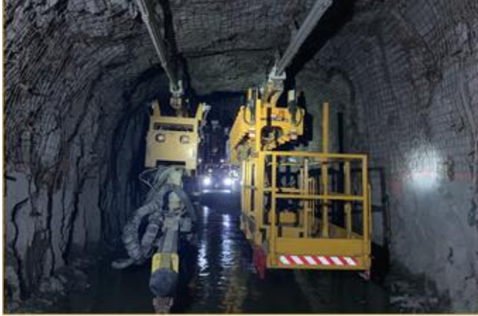
Two-way traffic via dual monorails
