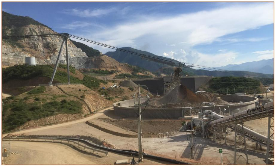
El Limon RopeCon and Guajes Crusher Stacker Conveyor Discharging SAG Mill Feed onto the Fine Ore Stockpile On the Right, the Dome being built over the Fine Ore Stockpile
